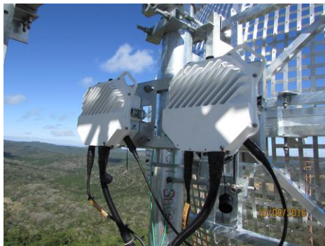
Figure 4 – BHP Site with 2+0 ODU and 1.20m Dual Pol Antenna. Figure 5 – BHP 1.20m Dual Pol Antenna
