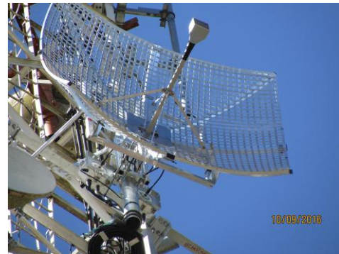
Figure 4 – BHP Site with 2+0 ODU and 1.20m Dual Pol Antenna. Figure 5 – BHP 1.20m Dual Pol Antenna
